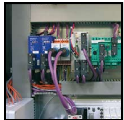
Remote-I/O-Schrank (Details)
