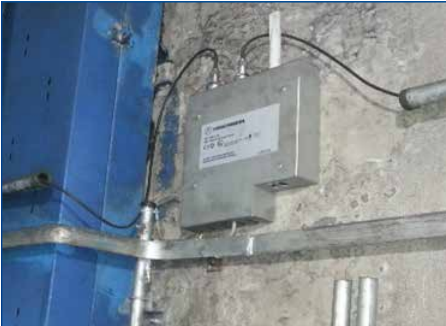
Industrial WLAN access points like this BAT300-F X2 are specially designed for hazardous environments and are approved for ATEX Zone 2 applications.
