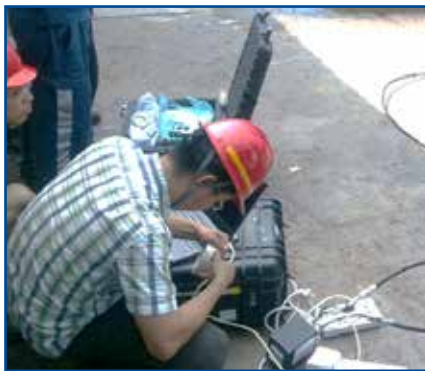
Belden experts were onsite to lead the installation process.
